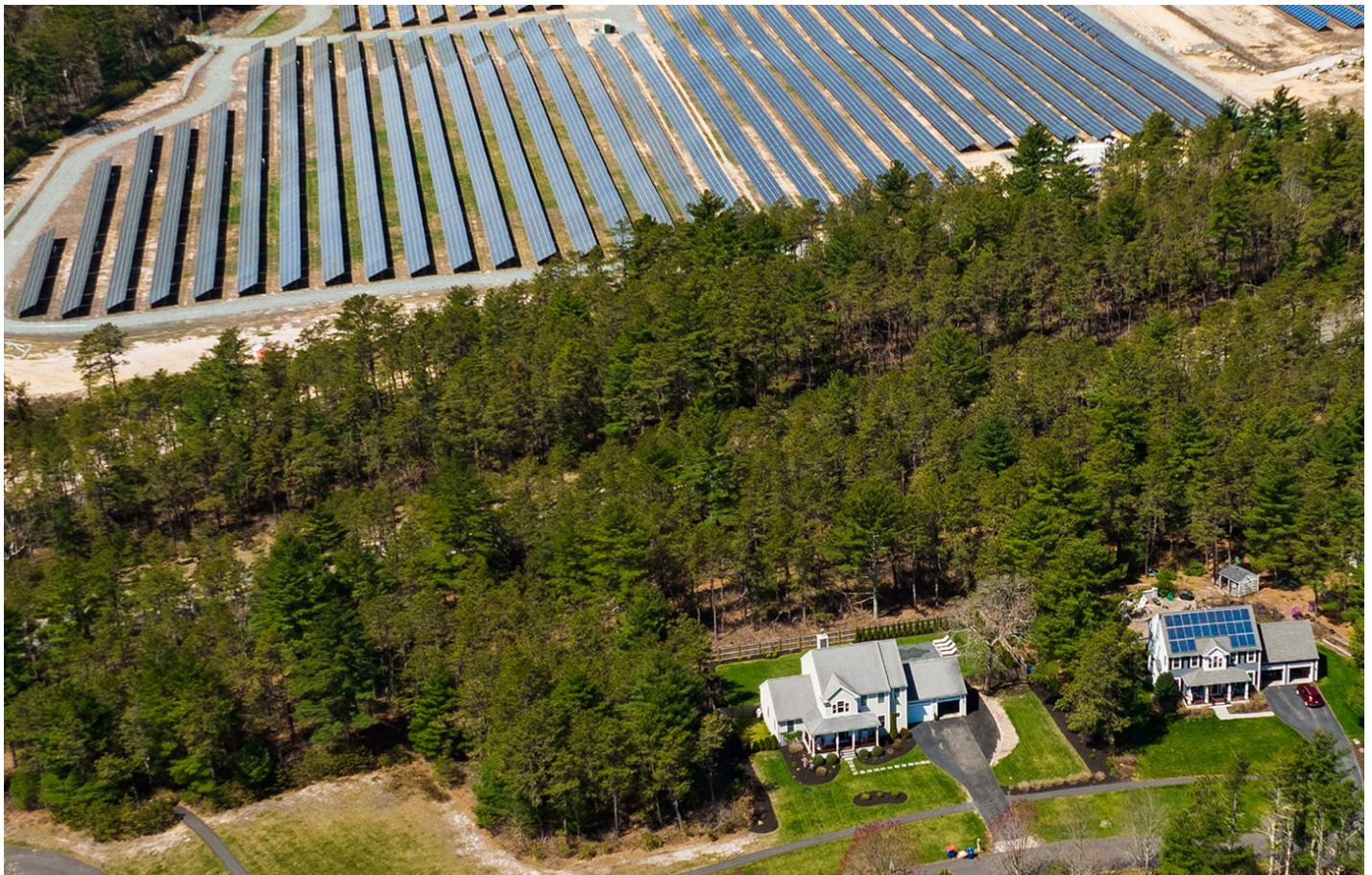
An A.D. Makepeace solar array in Wareham. ARAM BOGHOSIAN/FOR THE BOSTON GLOBE
